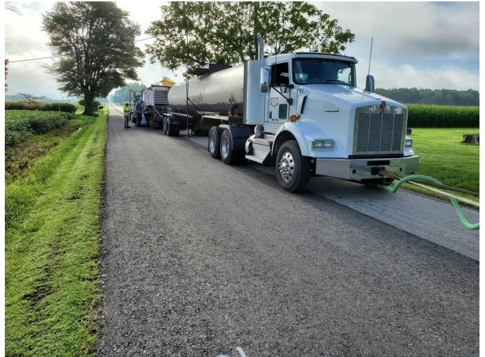
The Multi-Unit train processing Jackson Road
