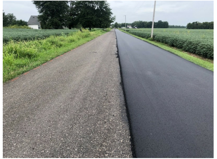
The 1.5-inch HMA surface and cured CIR mat
