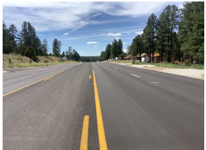
Completed project on SR-260 in Arizona
