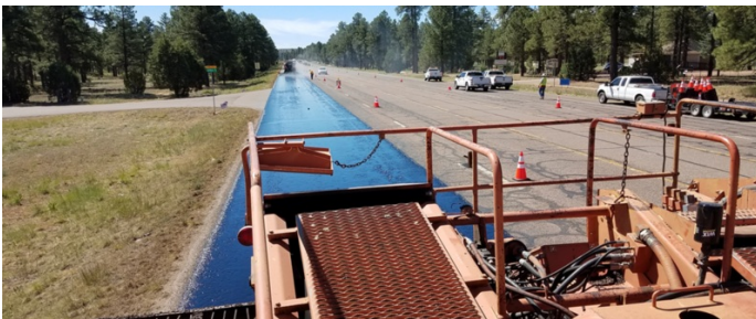
First course of the cape seal application in progress on SR-260.
