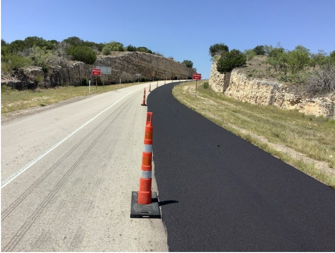
Micro Surfacing is being applied to Interstate I-10 in Ozona, Texas.
