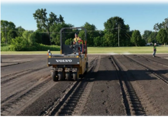
Compaction of FDR mix
