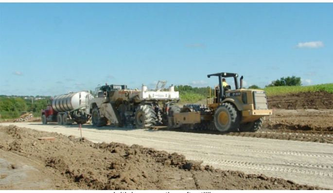
Initial compaction after tilling
