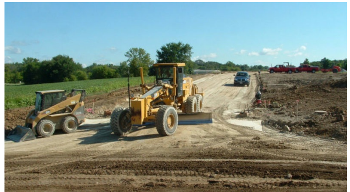
Final grading to elevation
