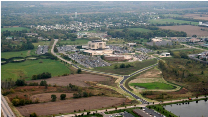
Aerial View of NIMC and new entrance road
