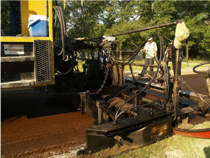
Micro surfacing is placed at the rate of about 22 pounds per square yard to produce a surface treatment between 3/8-inch and 1/2-inch thick.
