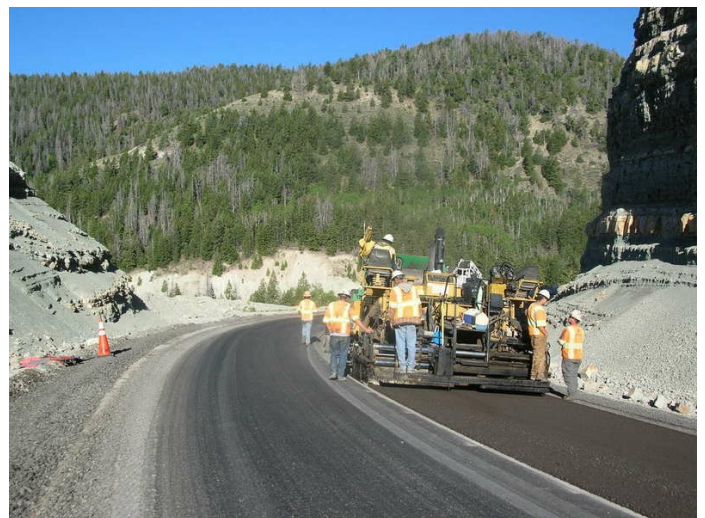
Burdick Materials Paving Operations Indian Canyon CIR
