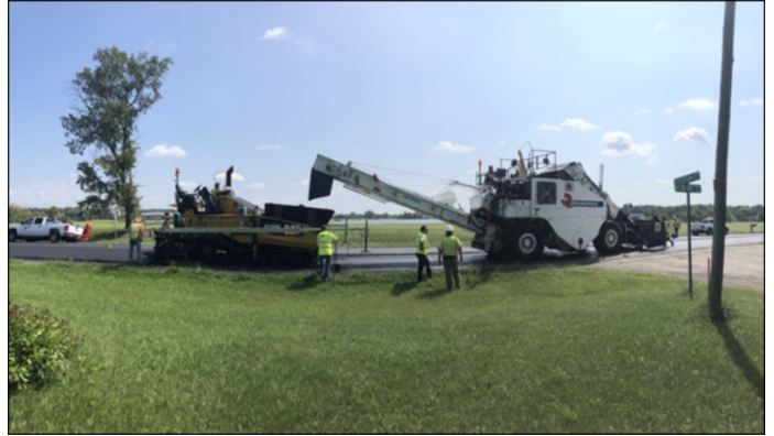
Paving of the 2.0-inch 12.5mm HMA surface
