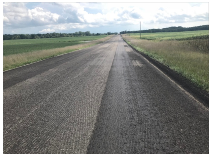
CCPR Mat after Profile Milling
