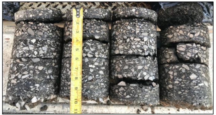
Pavement Samples taken during Investigative Sampling
