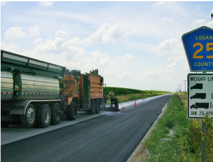
Applying the Microsurfacing
