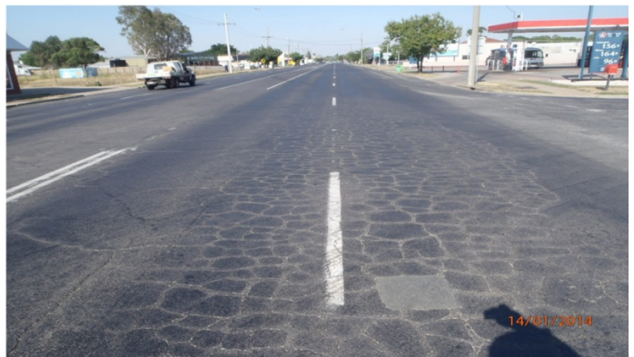
Pre-existing Condition - January 2014
