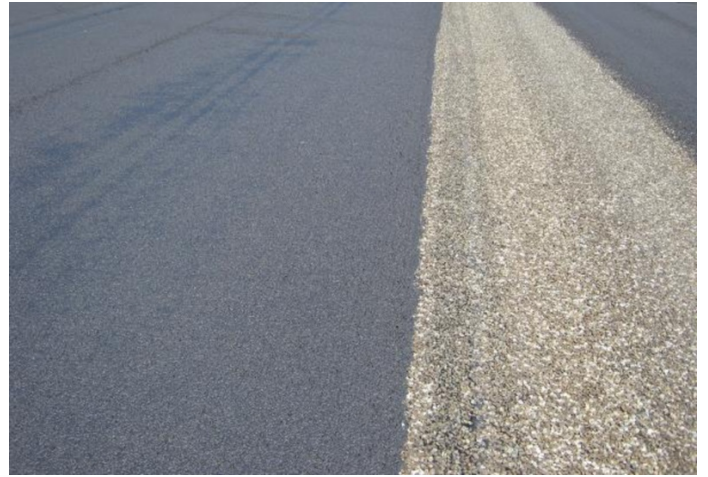
Installing the Micro Surfacing
