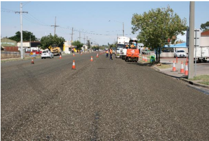
Installing the seal February 2014
