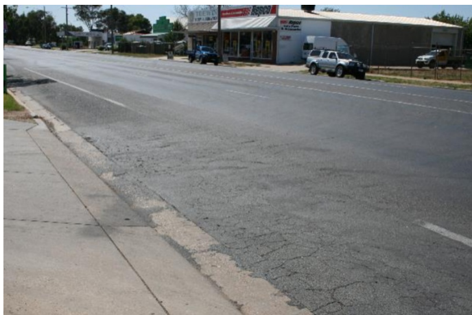
Pre-existing Condition - January 2014
