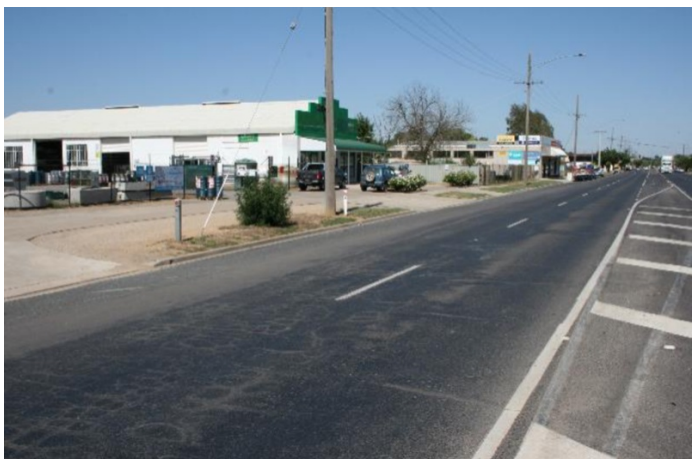
Pre-existing Condition - January 2014
