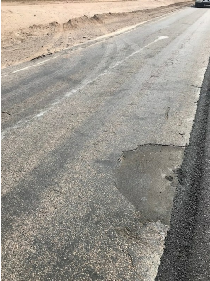
Existing Condition/ some patching
