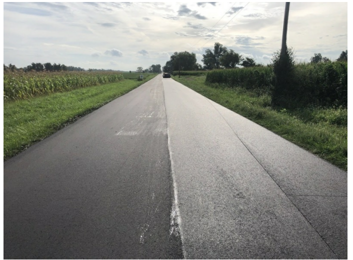
Finished 1.5-inch HMA surface on Jackson Road
