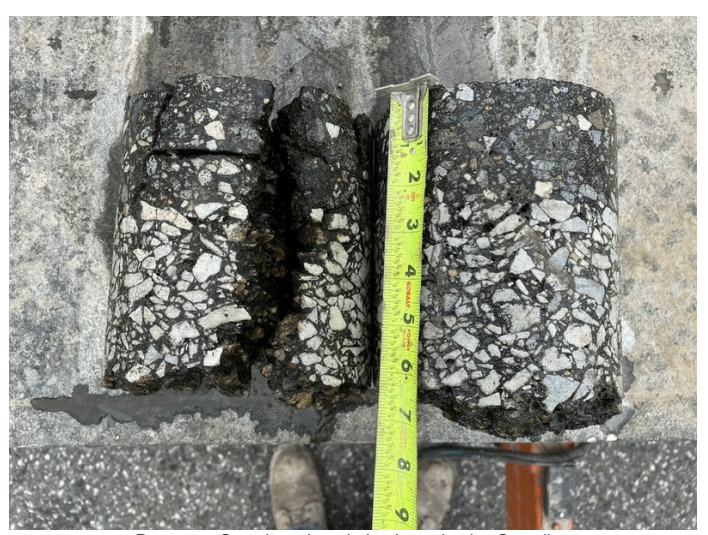
Pavement Samples taken during Investigative Sampling
