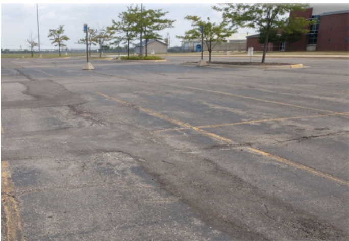
Parking lot prior to FDR
