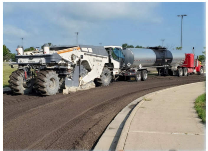
Performing FDR with emulsified asphalt
