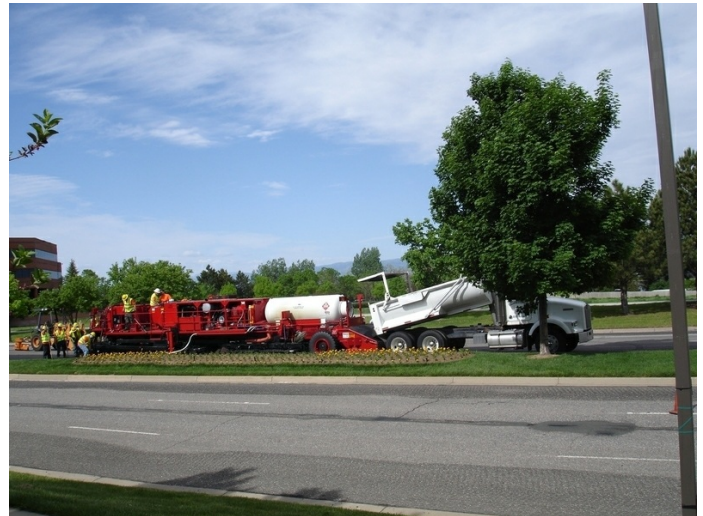
New hot mix asphalt produced in Denver's own hot mix plant is delivered to the Cutler Repaving equipment.
