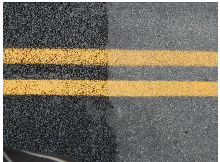
Finished Surface comparison - fiber reinforced interlayer with chip finish on right / PPST Overlay Finish on left
