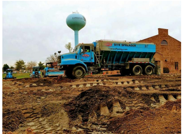
Applying and mixing Portland cement
