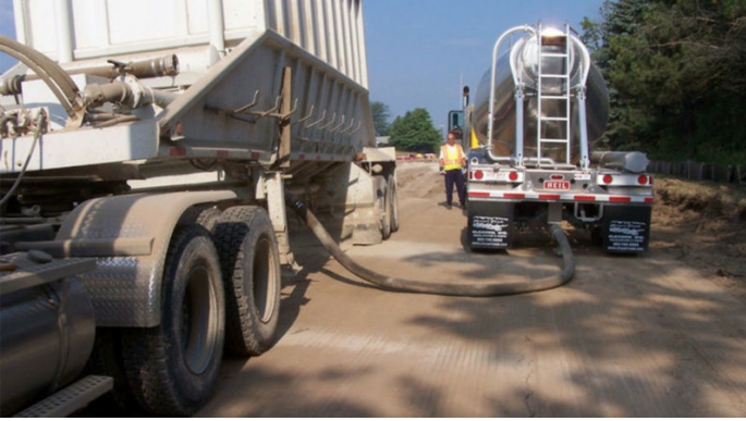
Pneumatic bulker loading spreader truck
