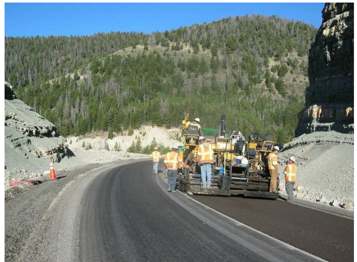
Burdick Materials Paving Operations Indian Canyon CIR
