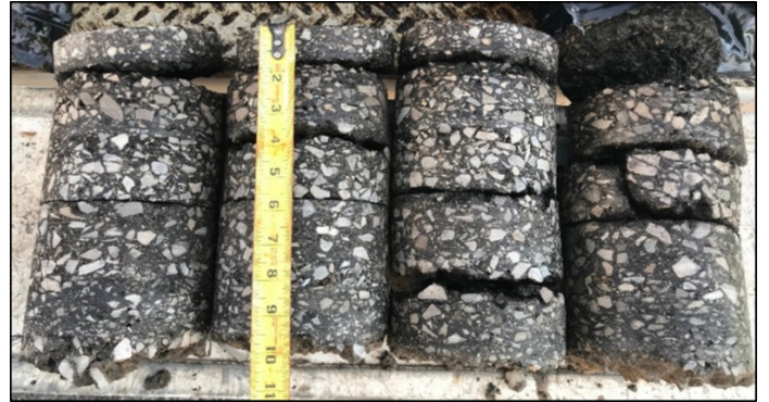
Pavement Samples taken during Investigative Sampling
