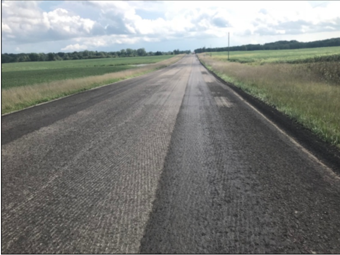
CCPR Mat after Profile Milling
