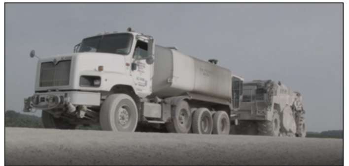
10.0-inch Cement FDR process
