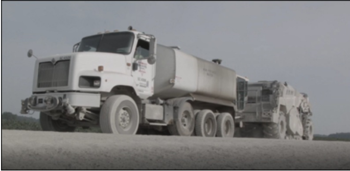
10.0-inch Cement FDR process
