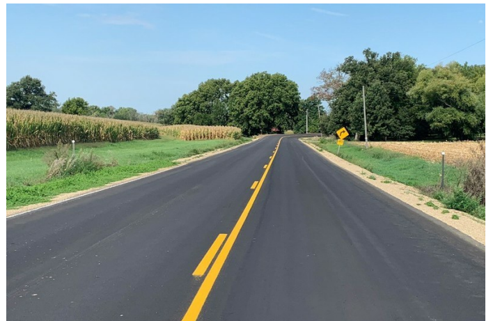
Finished Project with Cape Seal Surface
