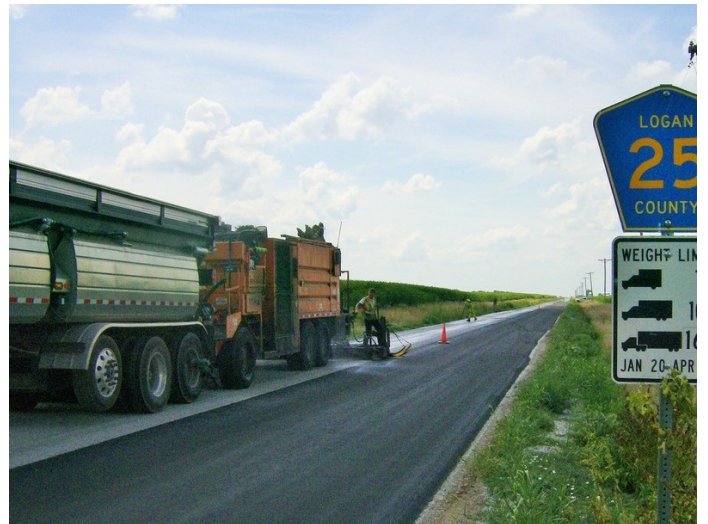
Applying the Microsurfacing
