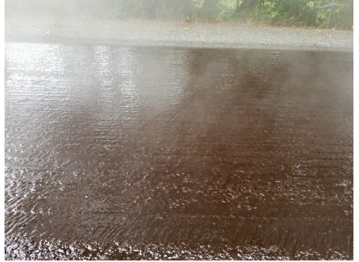
Freshly applied emulsion
