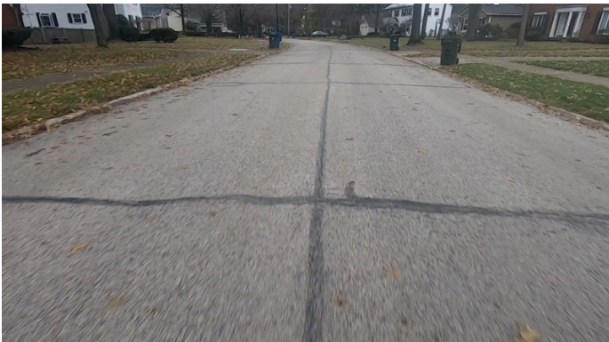
Roadway that Received a Crack Seal Treatment at the Right Time
