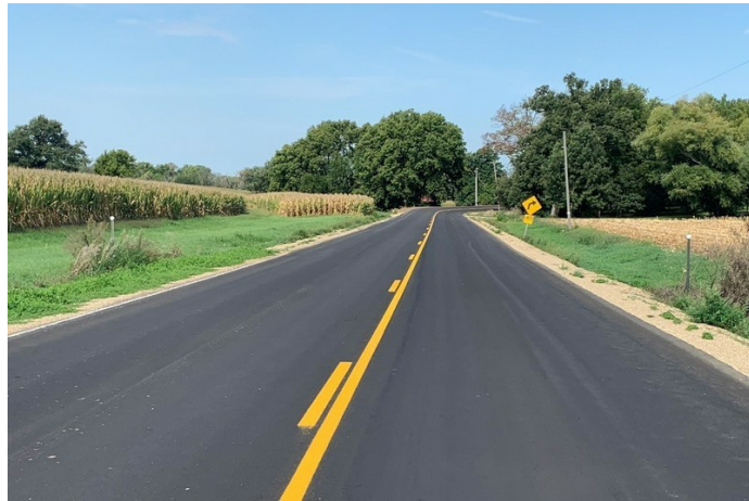
Finished Project with Cape Seal Surface
