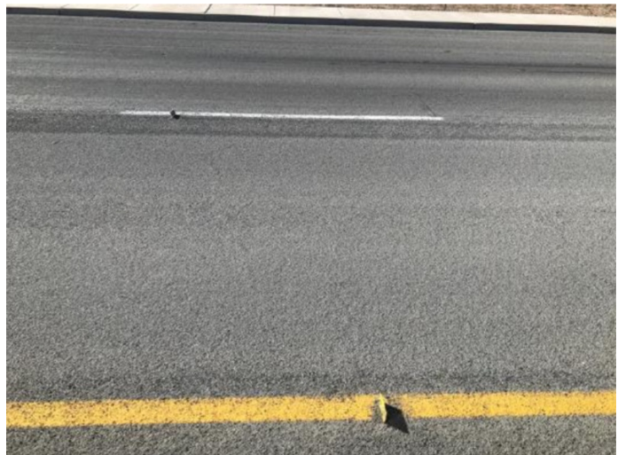
Completed Scrub Seal
