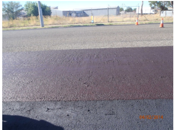
Installing the Micro Surfacing
