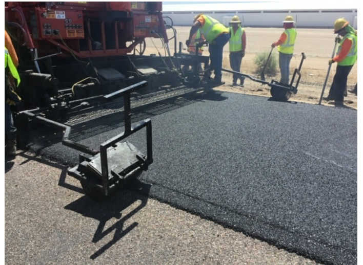
Final 1" recycled layer under 1" new layer AR.
