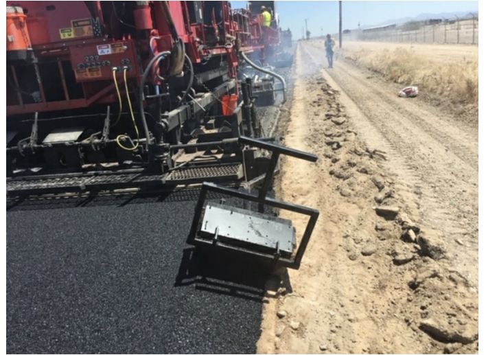
Hot in Place Repaving/safety edge
