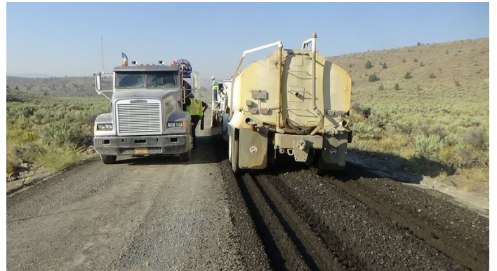
Keeping the road open during construction
