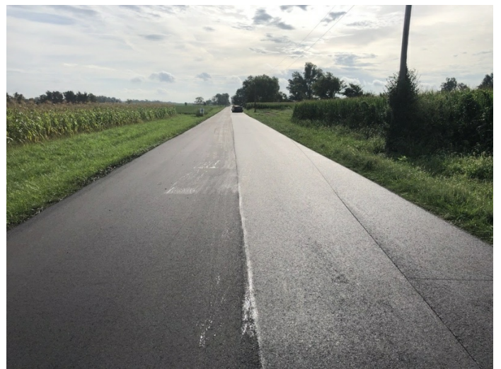
Finished 1.5-inch HMA surface on Jackson Road
