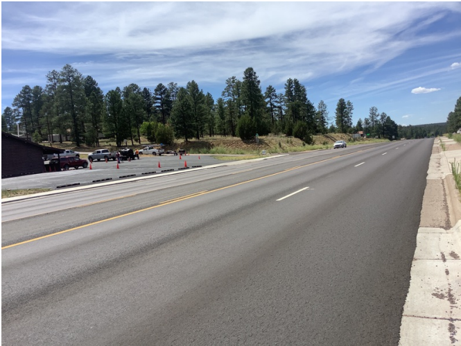
Crews wrap up this completed project on SR-260 in Arizona.
