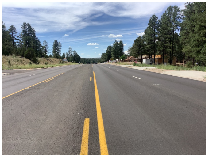
Completed project on SR-260 in Arizona
