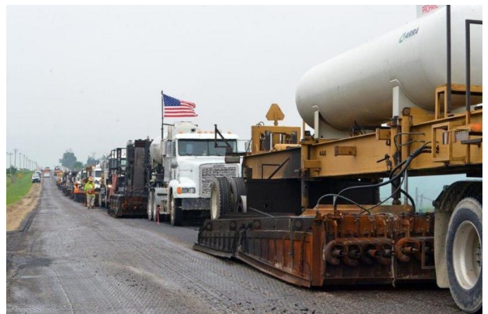
Performing 2-inch HIR on Sinclair Ave
