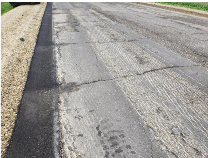
Sinclair Ave after profile milling
