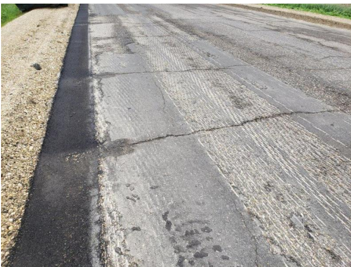
Sinclair Ave after profile milling
