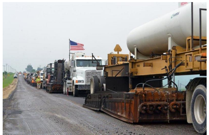
Performing 2-inch HIR on Sinclair Ave
