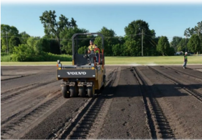
Compaction of FDR mix
