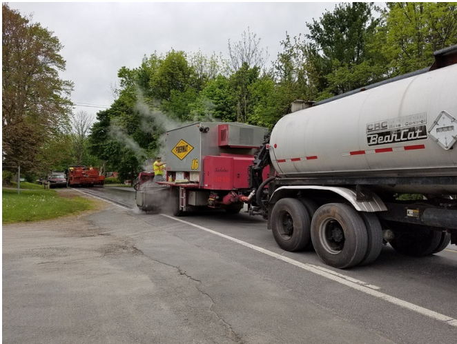
The Gorman Group laying interlayer fiber reinforced system
