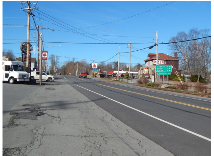
Lake Louise Marie Road finished with PPST Type B
