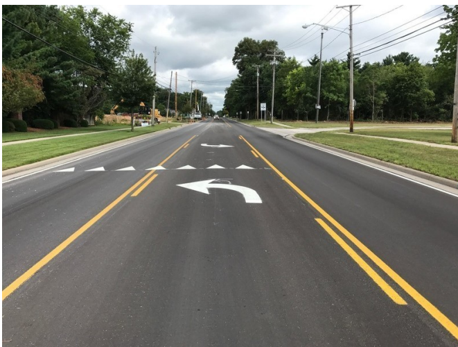
Micro surfacing in Sylvania
