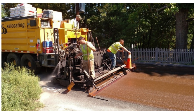
Application of Microsurfacing
