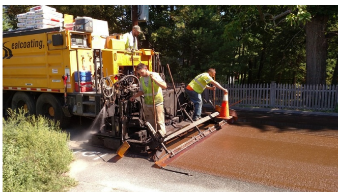
Application of Microsurfacing
