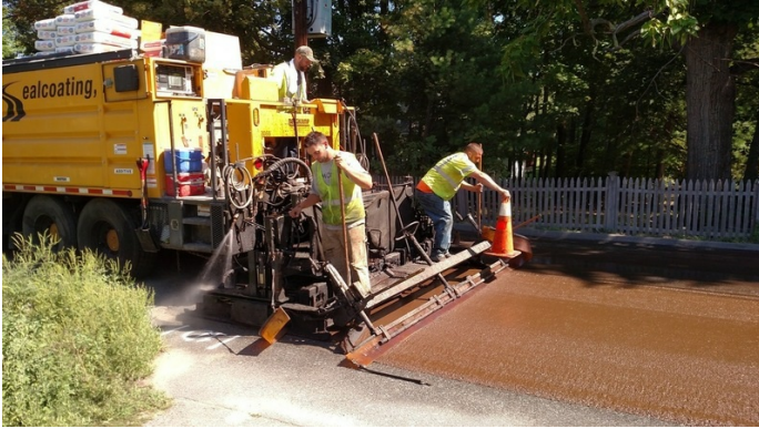
Application of Microsurfacing
