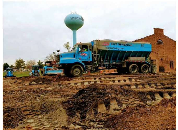
Applying and mixing Portland cement
