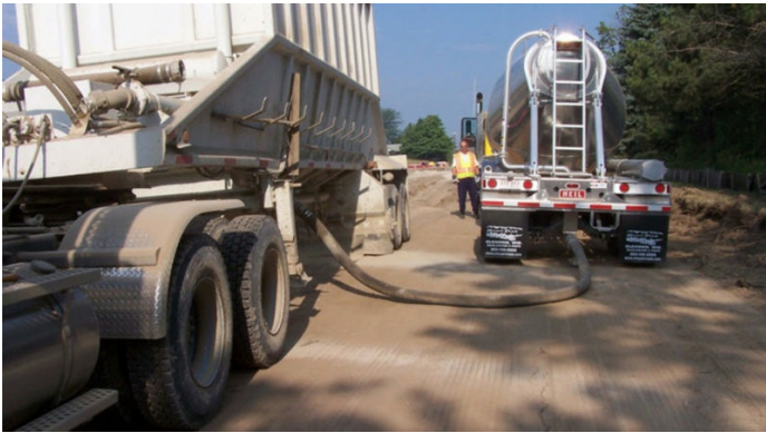
Pneumatic bulker loading spreader truck
