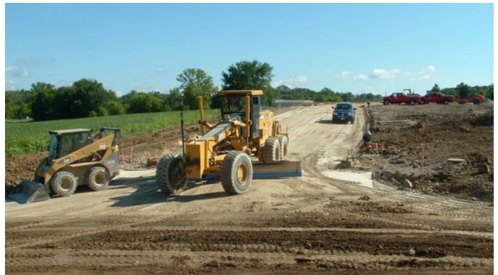
Final grading to elevation
