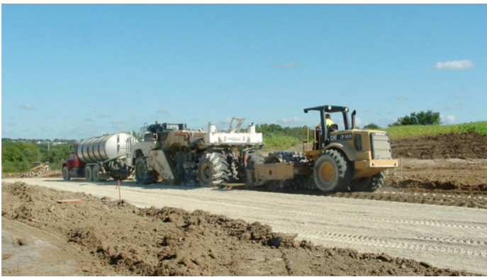
Initial compaction after tilling
