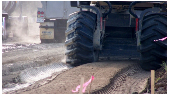
Uniformly tilled material
