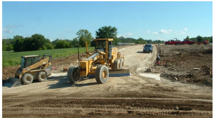
Final grading to elevation
