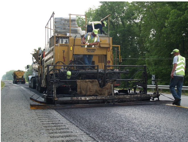
Micro Surfacing is applied over an entire 12-foot lane in a single pass.
