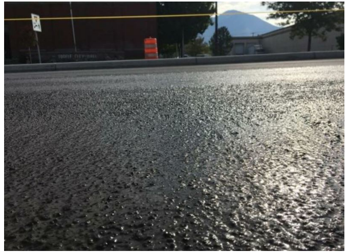
Close up of micro surfacing application
