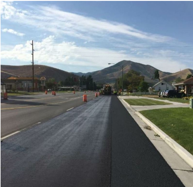
Micro Surfacing Application Intermountain Slurry Seal
