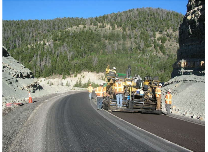
Burdick Materials Paving Operations Indian Canyon CIR
