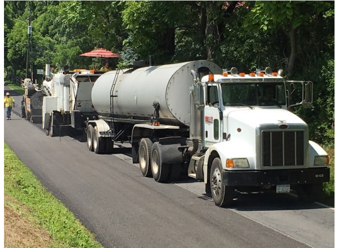
Cold-In-Place Recycling "train" with tanker of CSS1-h emulsion hooked onto milling machine.
