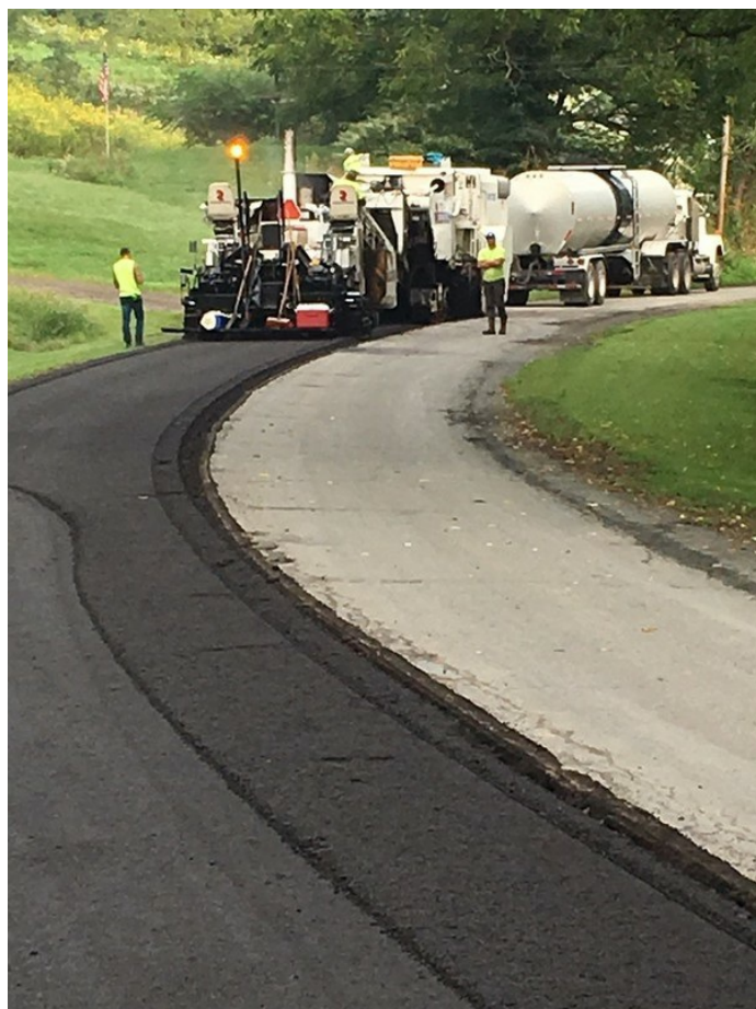
Cold-In-Place Recycling "train" with tanker of CSS1-h emulsion hooked onto milling machine and paver.
