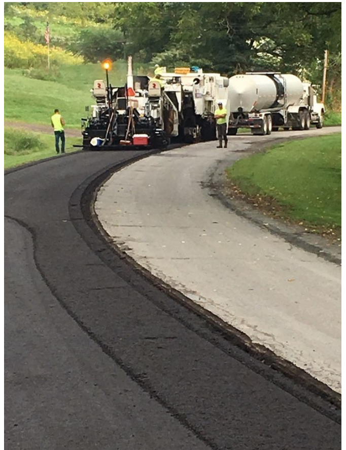
Cold-In-Place Recycling "train" with tanker of CSS1-h emulsion hooked onto milling machine and paver.
