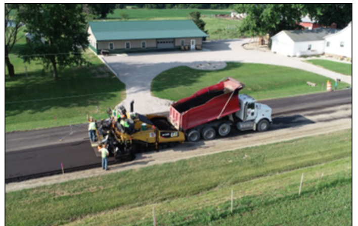
Paving of the 6.0-inch CCPR lift
