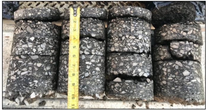
Pavement Samples taken during Investigative Sampling
