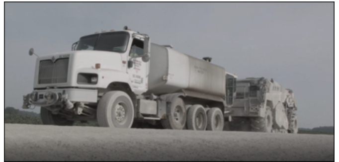
10.0-inch Cement FDR process
