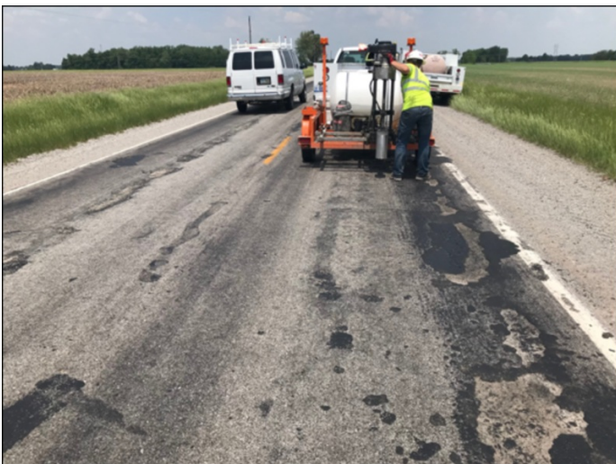
Existing Pavement Surface during Investigative Sampling
