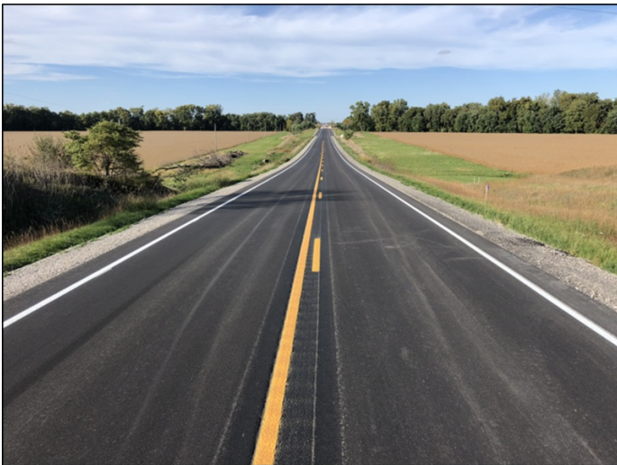
Final pavement surface
