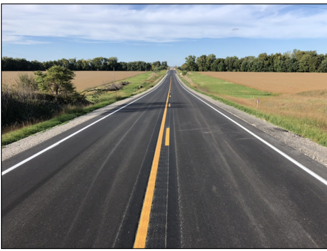
Final pavement surface
