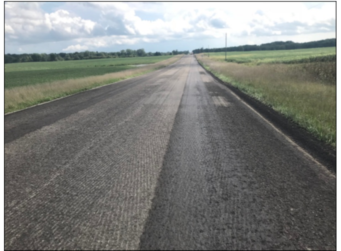
CCPR Mat after Profile Milling
