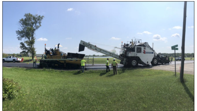
Paving of the 2.0-inch 12.5mm HMA surface
