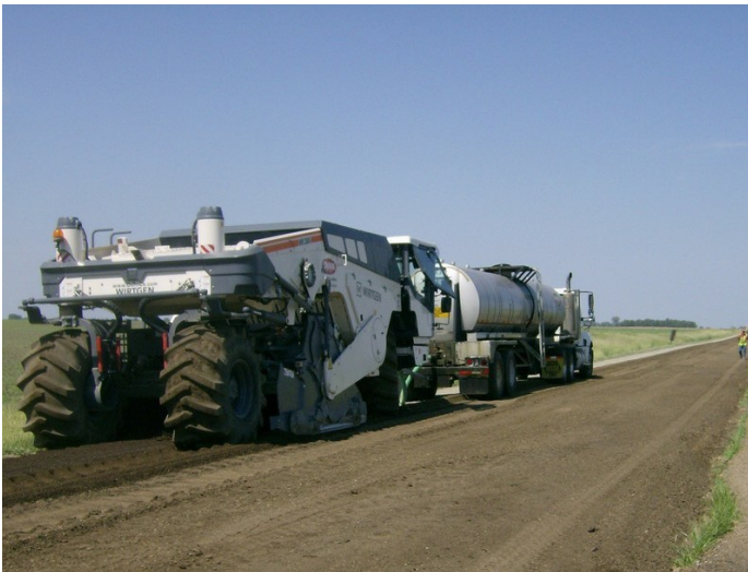
FDR Stabilization with Engineered Asphalt Emulsion
