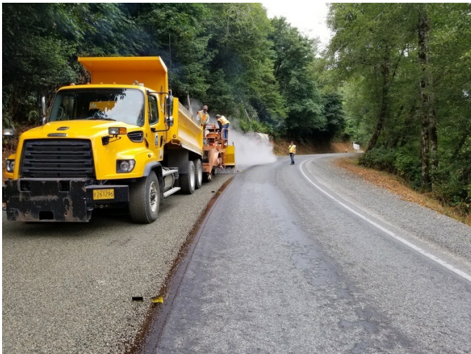
Chip seal in process
