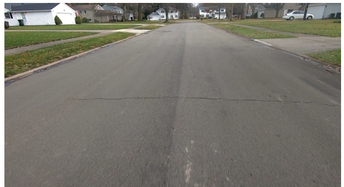
Upcoming Crack Seal Candidate
