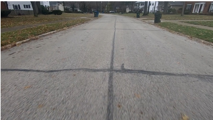
Roadway that Received a Crack Seal Treatment at the Right Time
