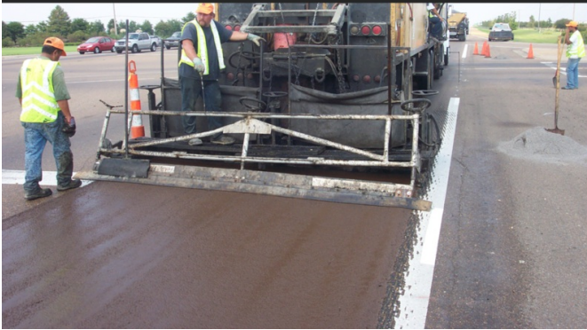
Photo Recap 2005 Micro Surfacing Application
