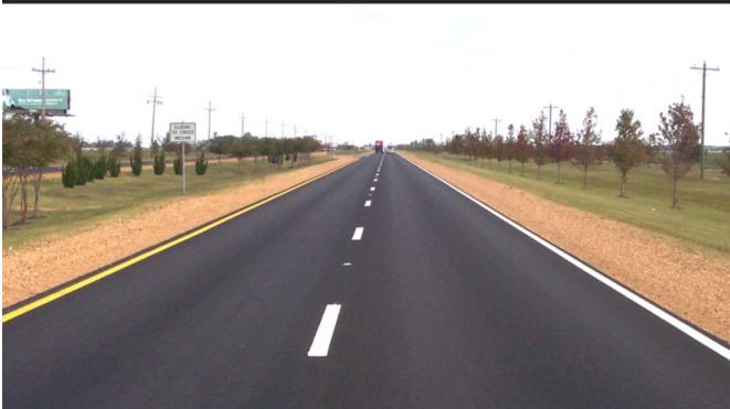
Photo Recap 2005 After Micro Surfacing Application
