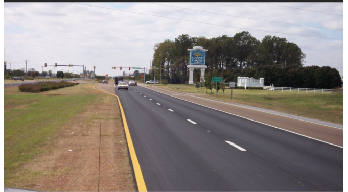
Photo Recap 2005 After Micro Surfacing Application
