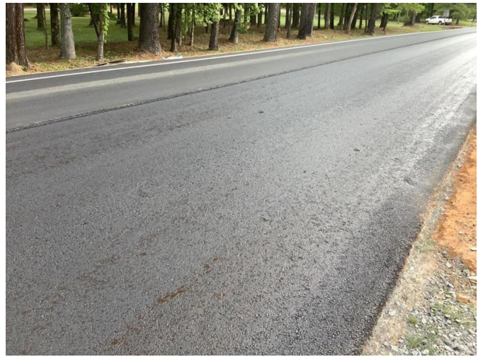
Broken Tack (Uniform Coverage)
