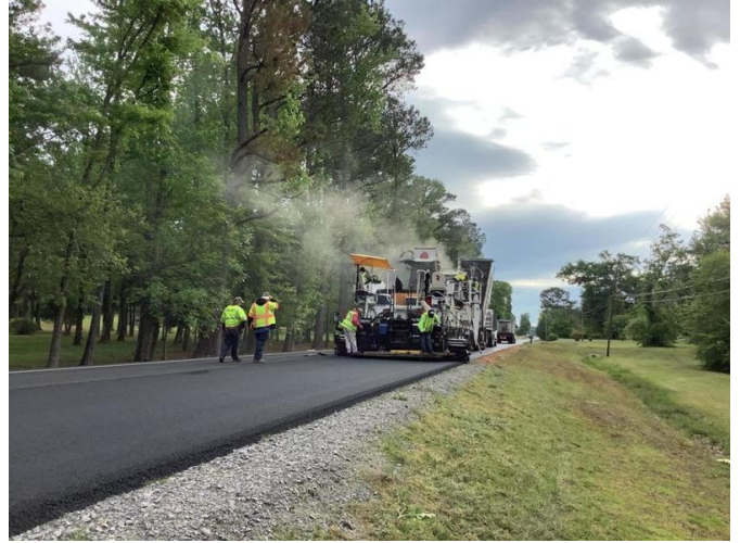
Paving Hot Mix
