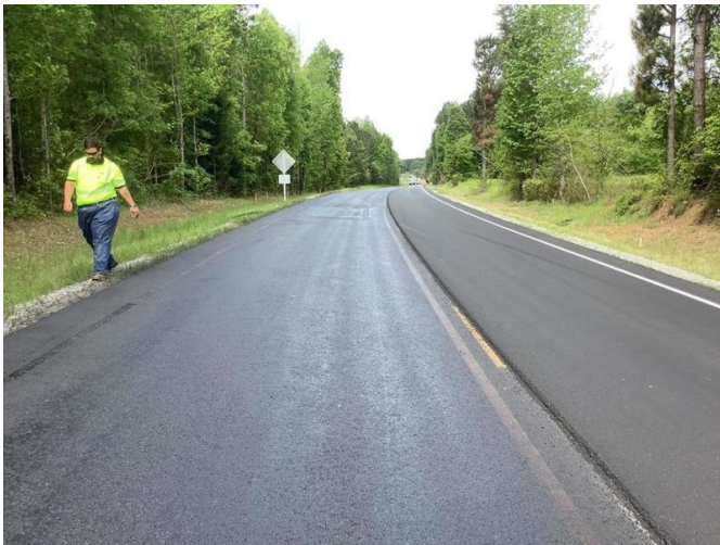
Perfect Uniform Coverage of Broken Trackless Tack
