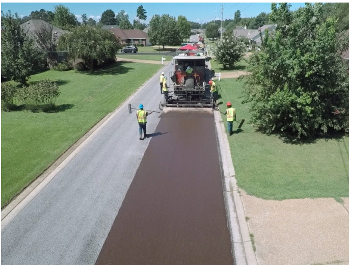
Chip Seal and Microsurfacing was applied to this neighborhood in Rankin County
